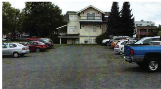
348 WESLEY STREET EXISTING THREE STOREY OFFICE BUILDING
